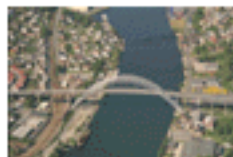
Fredrikstad bridge from the south.
